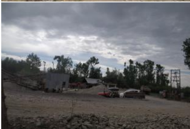
Stone Crusher unit near sadoora Project site from Kamad side
