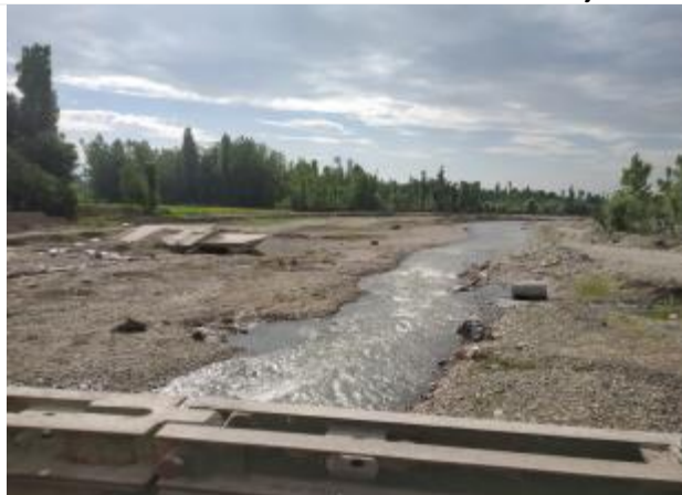
Downstream side of Brinji Nallah at Sadoora
