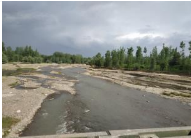
Upstream side of Brinji Nallah at Sadoora
